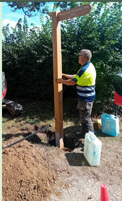
A fingerpost being installed
